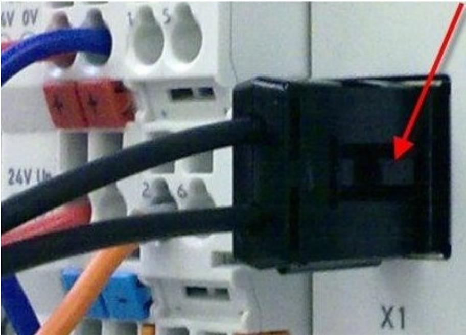
Fig. 28: Latching lug with release catch on the POF duplex plug
